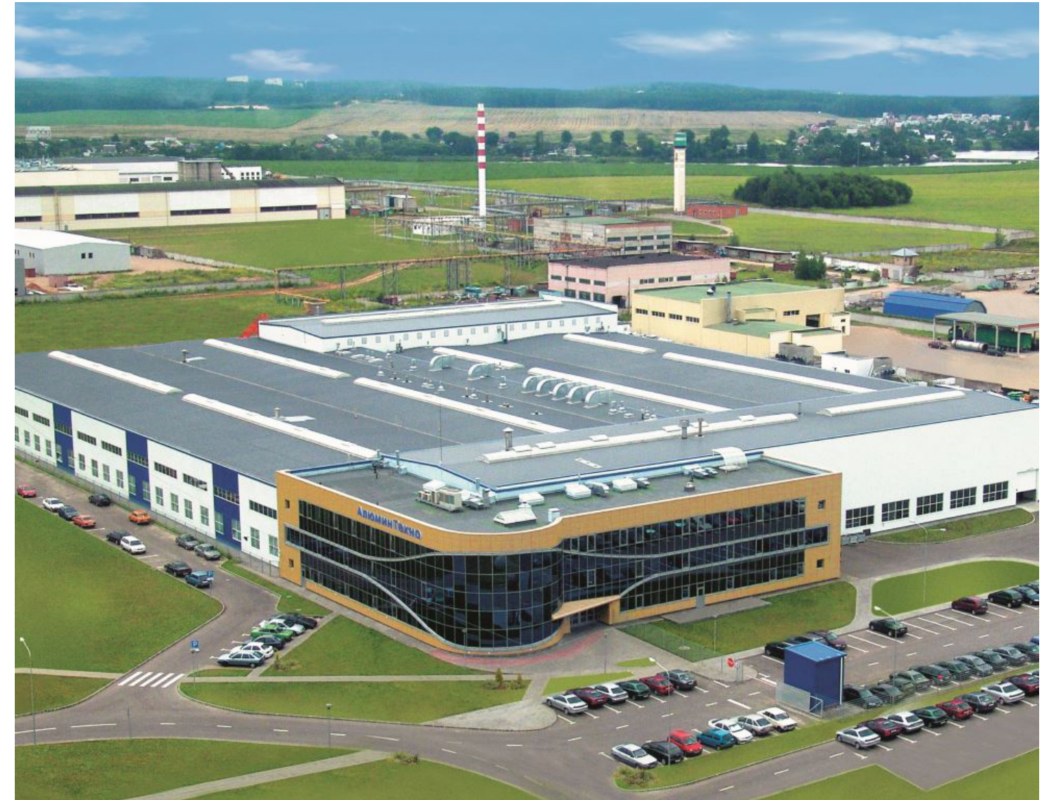
AluminTechno, LLC Production Facility
